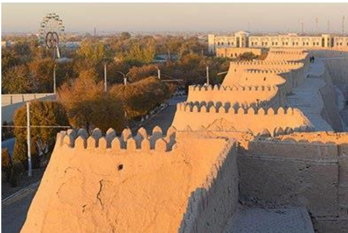
Picture 2. Khiva. View from the top of citadel to the new development.
